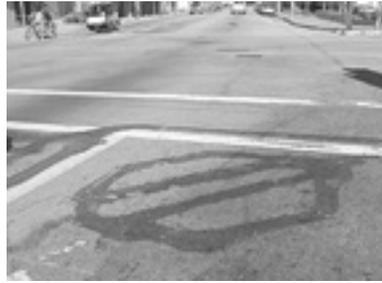
**Loop detectors** work basically like metal detectors. They consist of several “wraps” of
