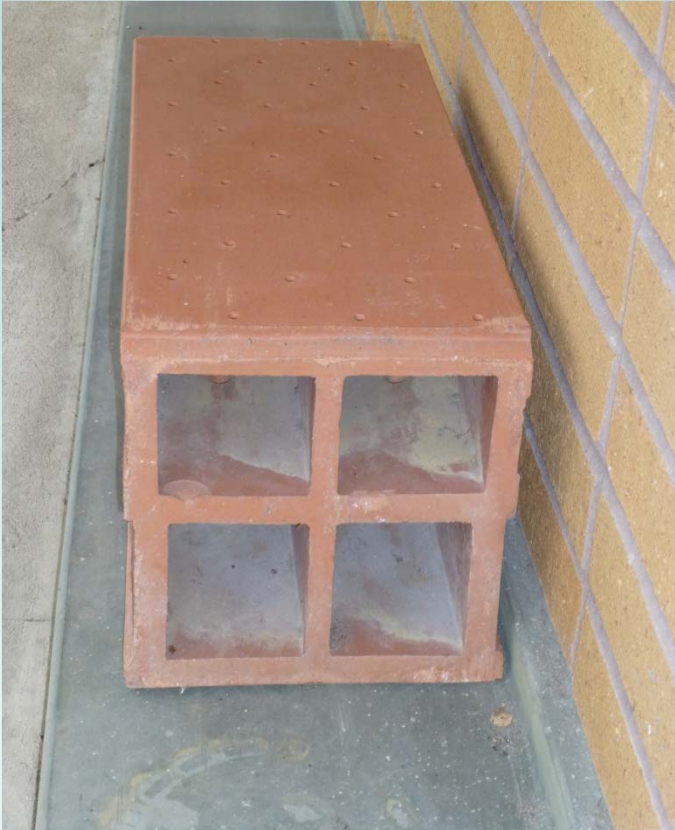
Clay Tile Underdrain
