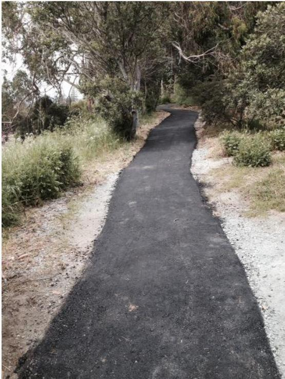
decomposed granite material to asphalt. The pathway winds up East Cliff up to Ocean View, connects at the bottom with San Lorenzo. The new paved pathway is approximately lineal feet 1,000, and nearly 3,000 square feet of paving. Phase 2 is envisioned to be a spur trail that comes down from the Ocean View Park art station (earthquake debris which was converted to art) and will be another 540 lineal feet, or 1,600 square feet of paving.
