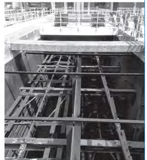
A flocculator undergoing rehab
