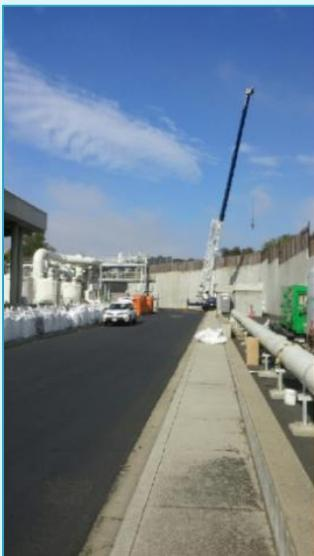
We completed the activated carbon exchange for carbon scrubber units #1 and #2. The carbon scrubbers provide a last polishing step in treating process foul air before releasing to the atmosphere.
