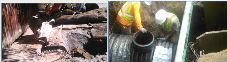
Crews are working in the Eastside and Seabright zones cleaning and inspecting sanitary sewers. This is part of our annual maintenance requirement to the system that occurs every 12 to 16 months.
